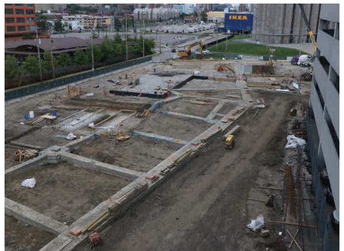
4210 Duncan construction in early 2020. Photo by Cortex staff.
